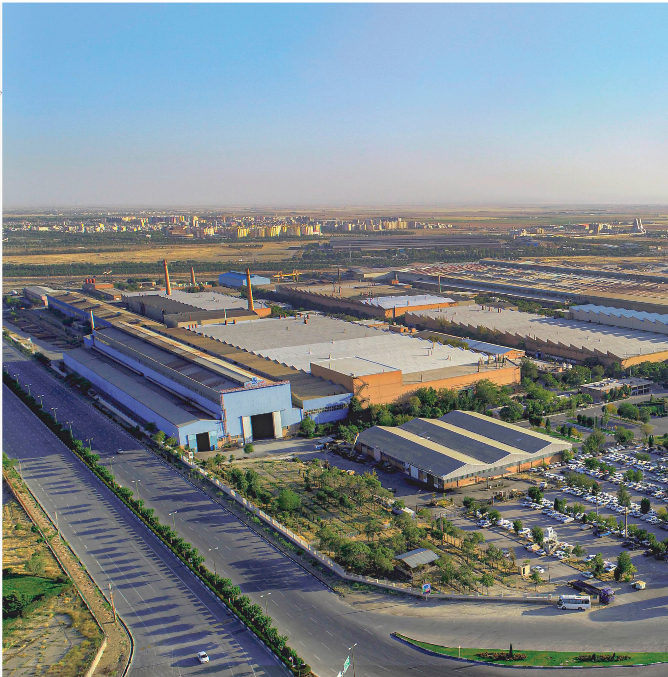
Top view factory Machine Sazi Arak
